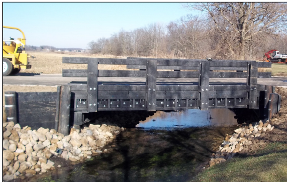
Bridge 174-0.56 over the Onion Ditch
